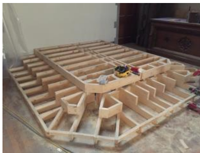
Chapel restoration progress
